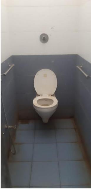
Specialized toilets for PWD
