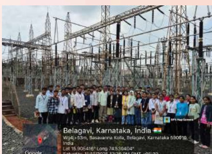
220 KV Switching Station, Kanabargi on 11th October 2025
